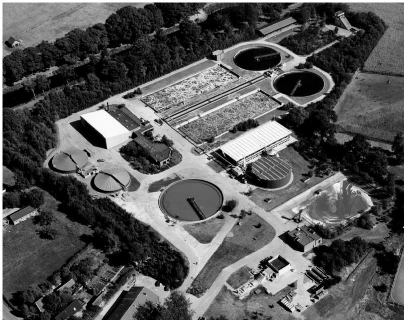
Fig. 1.3. Full-scale UASB plants (rectangular and circular installations in the center part of the photo) treating the combined reuse paper wastewater of three factories, and conventional aerobic post-treatment (right upper part of photo) and micro-aerobic biogas-treatment facilities (in a small separate building positioned between the AnWT-installations) in the city Eerbeek, Netherlands.
